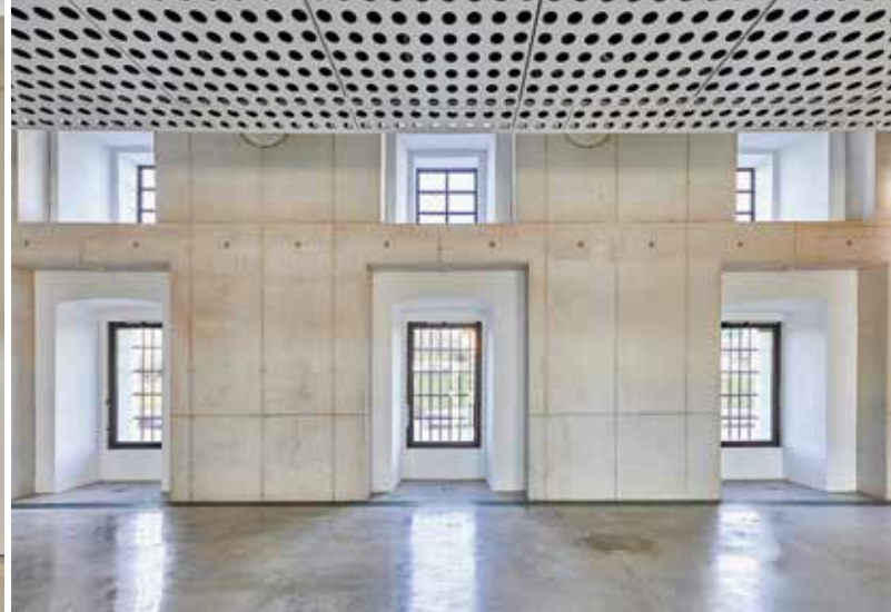
Inside, a reinforced concrete wall has been placed in front of the existing facade.
